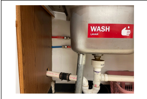
Photo No. 7 GZ-24: New Kitchen Sink Piping
